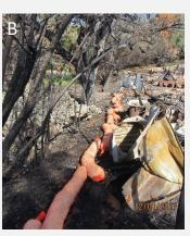
Figure 3. A) Water Board and Sonoma Ecology Center Staff collecting baseline samples at Sonoma Creek. Photo by Melissa Roberts, Sonoma Ecology Center. B) Erosion and drainage controls installed next to burned structure near creek.
